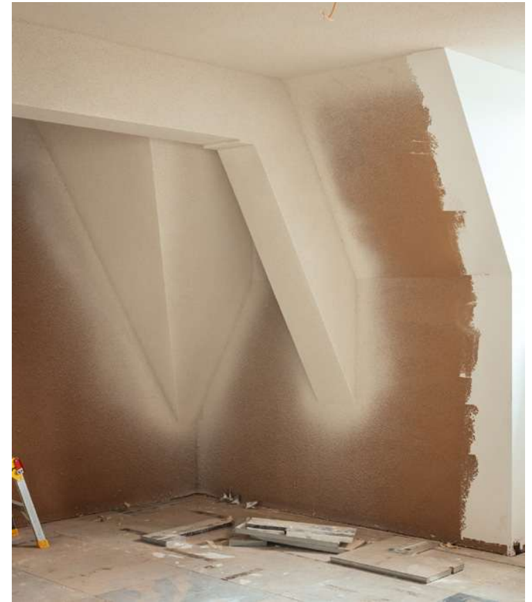
Walls sprayed in Cork
