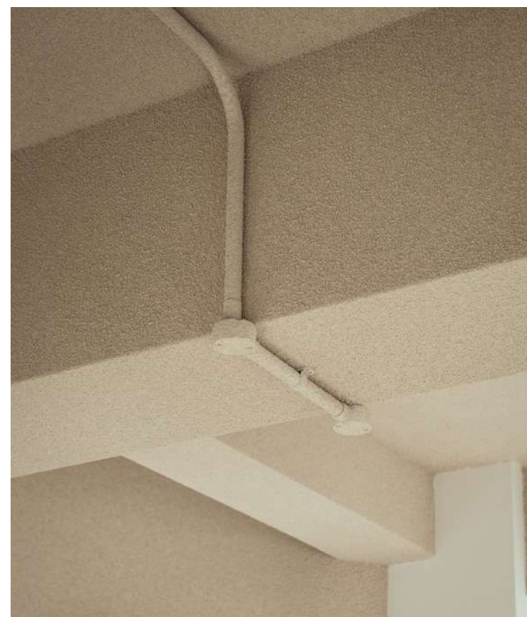
S4 completed SprayCork finish on soffit
