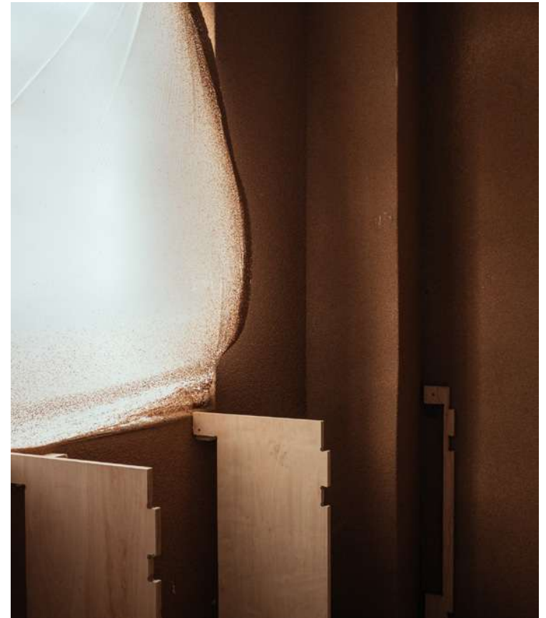
Walls sprayed in Cork
