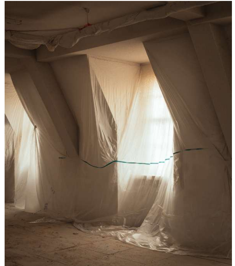
Walls sprayed in Cork
