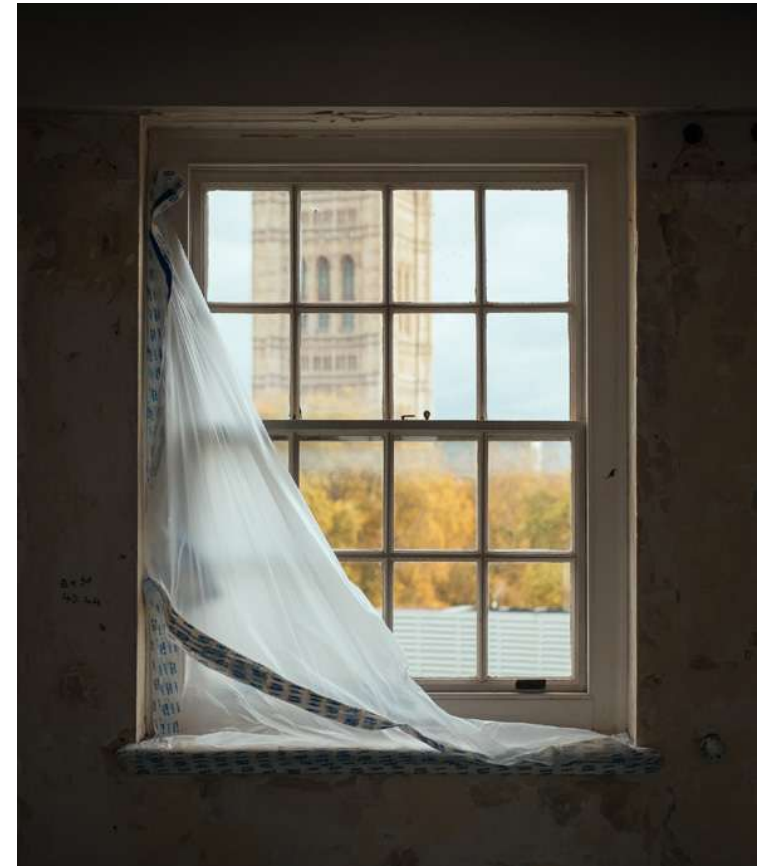
Office space during refurbishment
